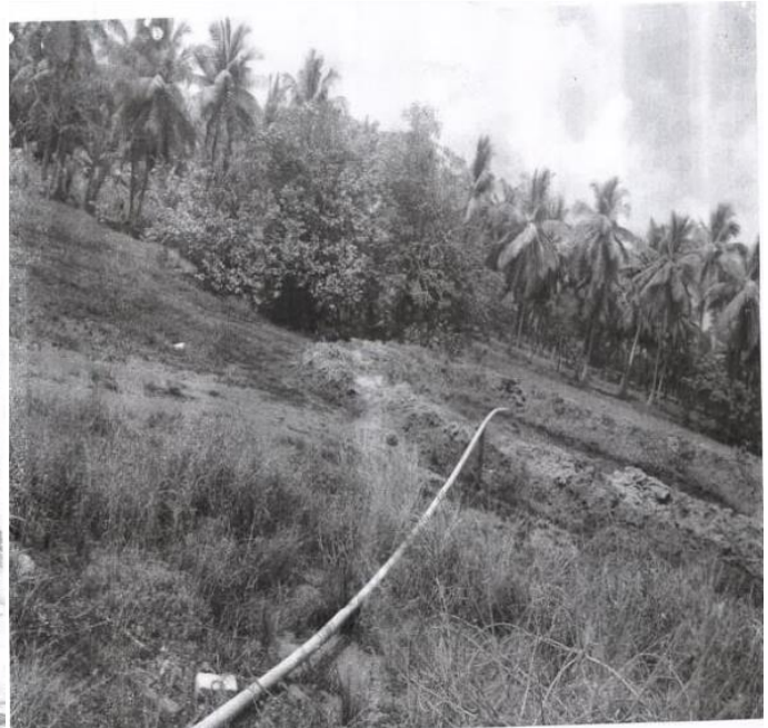
Flow Line to Waste Pit
