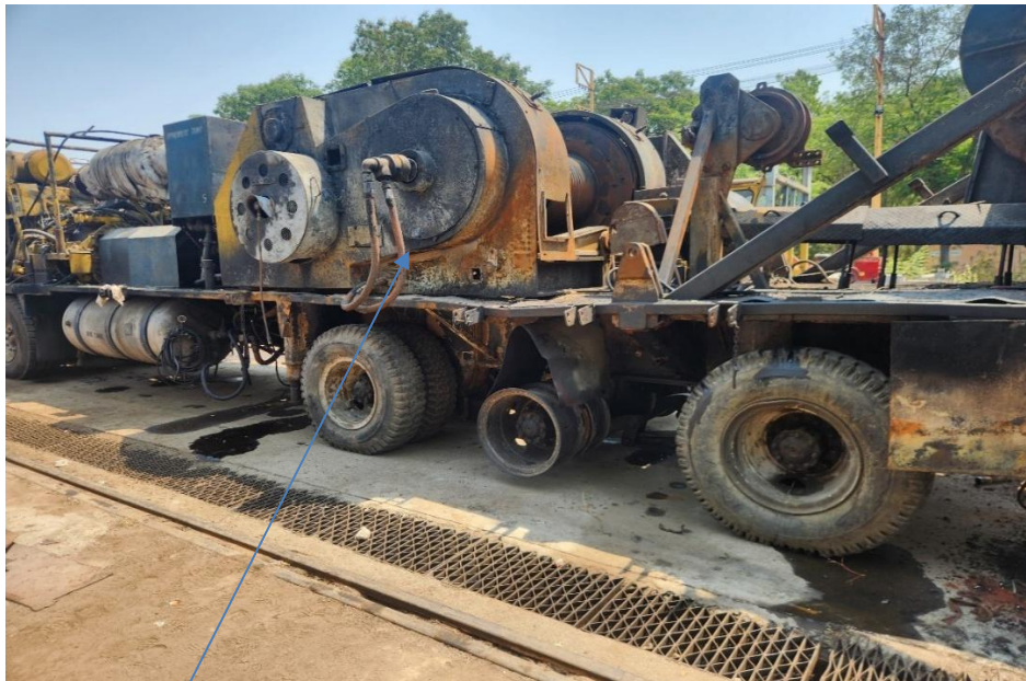
Draw works condition after fire
