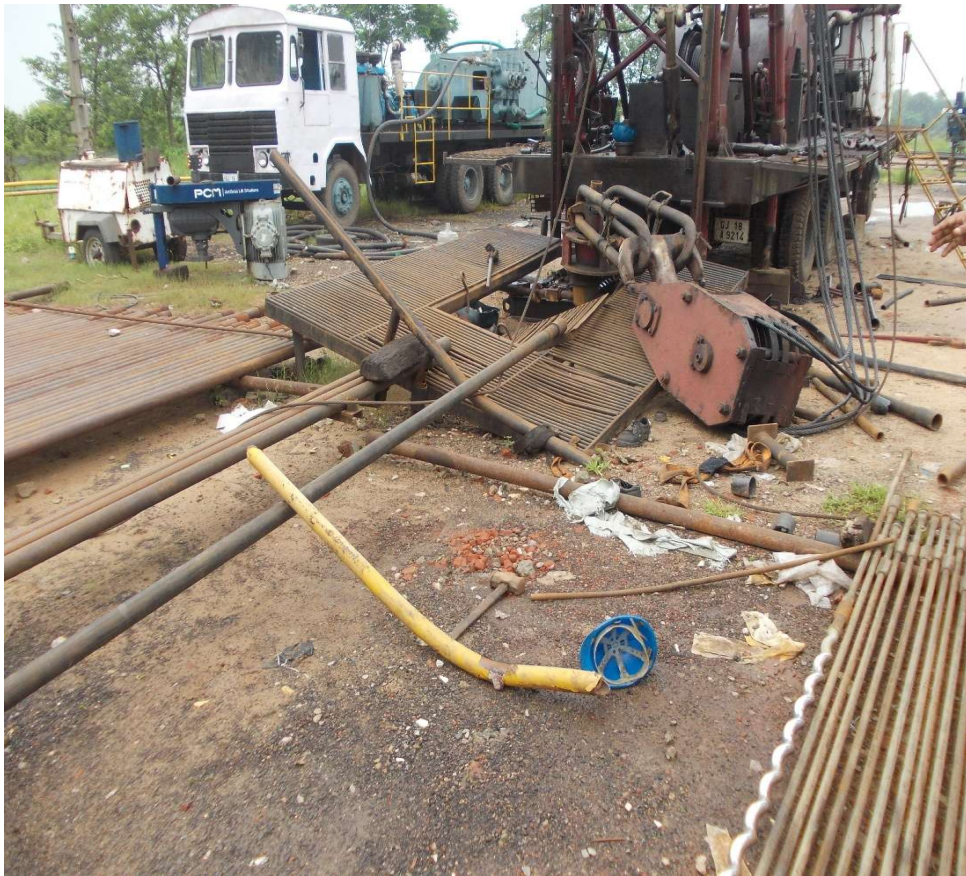
Photograph of Incident location
