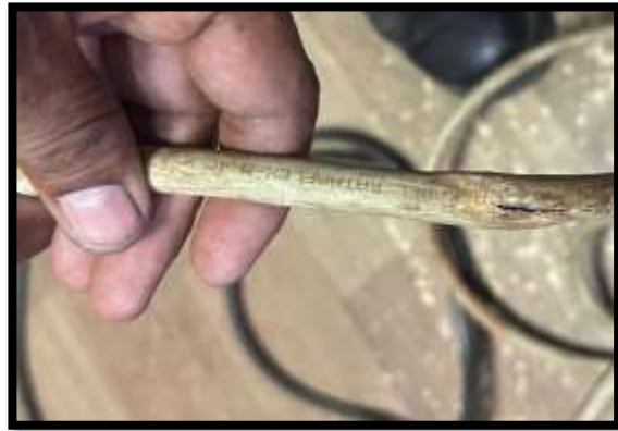
Temporary extension Box and cable
