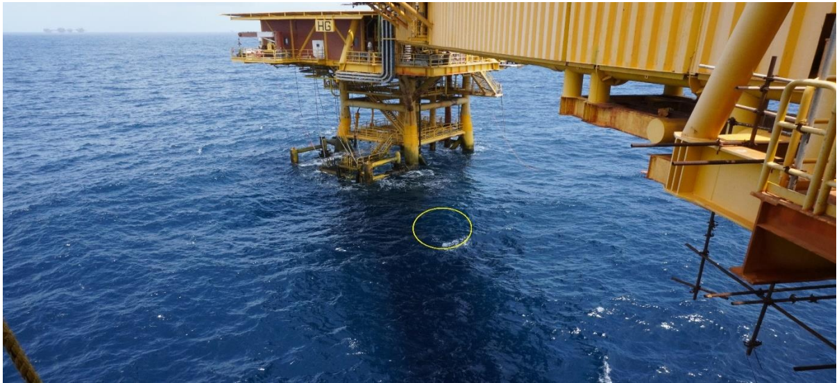
Photograph of Incident location
