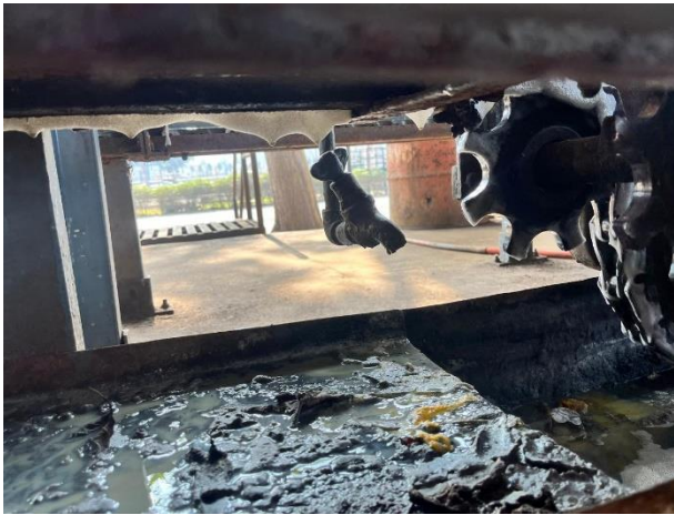
Isolation valve position
